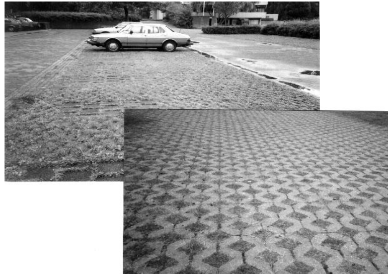
(a) : Example of block-reinforced grass used for vehicle hard-standing areas
